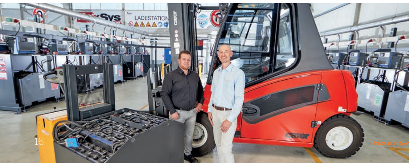
Managing Director Heino Hövelmann (right) and General Logistics Manager Michael Michailidis explained the benefits of the new battery charging station at RheinfelsQuellen. In the foreground is a four-tonne battery block for the electric forklift.
